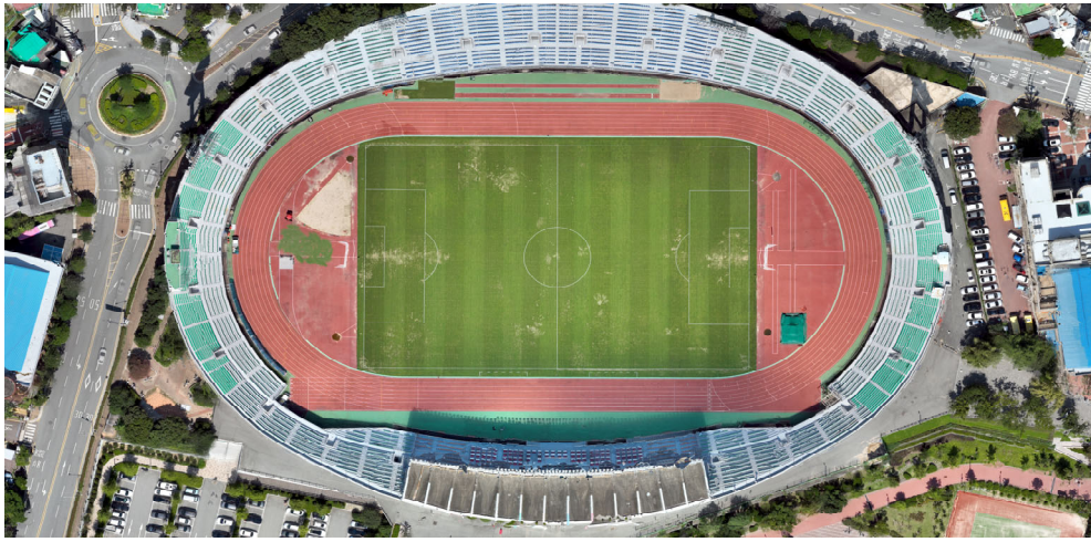
Fig. 3. UAV-based orthomosaic of the primary study site, Gudok Stadium.
